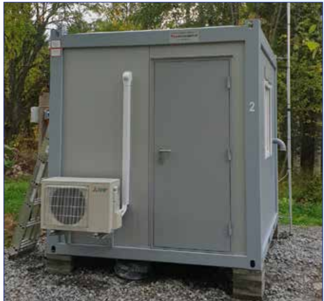
Fig. 22 The new measurement container on its gravel foundation at the Pötsönvaara air quality monitoring station. The sample air inlet line can be seen close to the right-hand side back corner. An air-source heat pump, capable of cooling the container in summer, is beside the container door.
