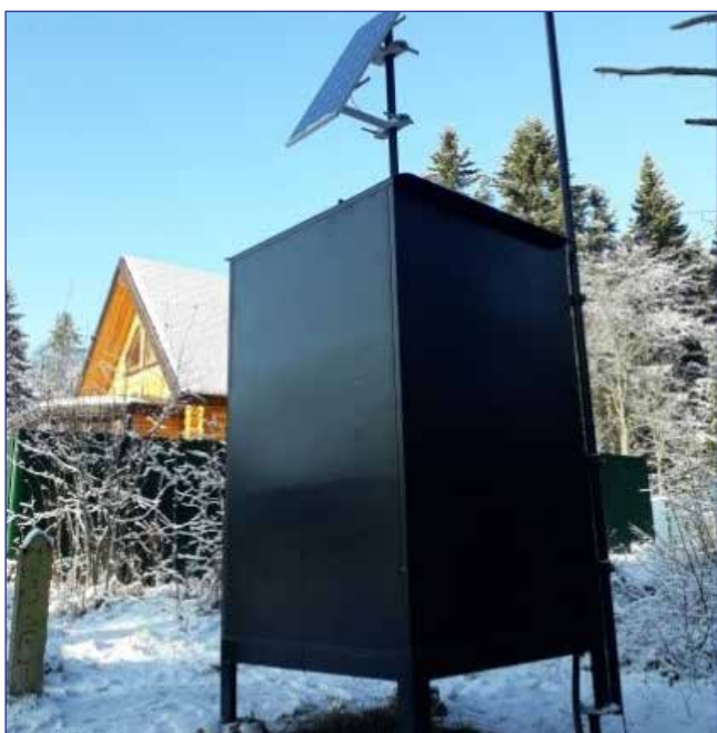
Fig.12 AHCC at the Uuksunjoki river – Uuksu settlement
